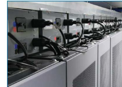
Plug-in units are offered with a wide variety of receptacles, circuit breakers, and drop cords. Multiple circuit breaker plug-ins are offered and can be used in high-density applications.
