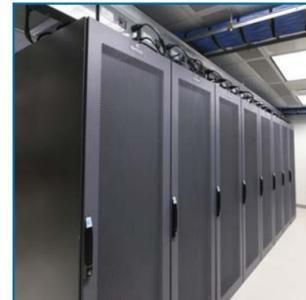
The 225 Amp STARLINE supplies power to rows of computer cabinets used in data centers and for development, testing, and manufacturing of computer networking equipment. It replaces hardwired raceway with bulky, fixed position outlets.
