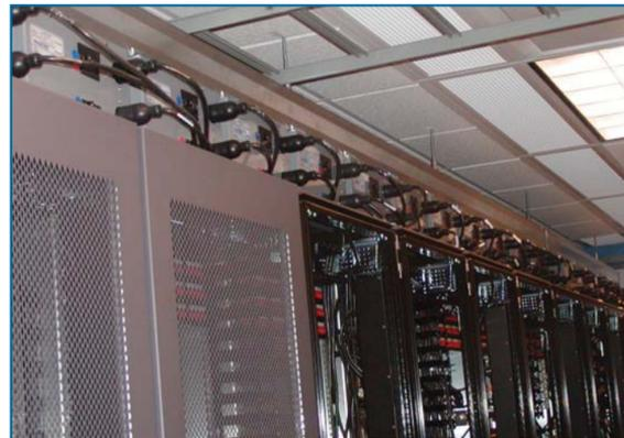
4 copper conductor, 3-circuit Starline Track Busway is available with 100, 160, or 225 Amp busbars, 200% Neutral and Isolated Ground.
