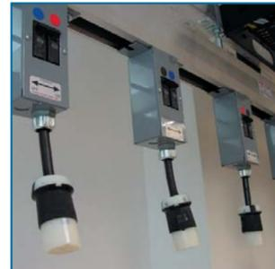
Each power module is circuit protected with circuit breakers or fuses right at point-of-use.
