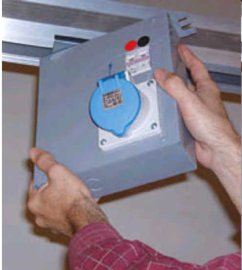
Figure 9 – Busbar Tap Box Install
